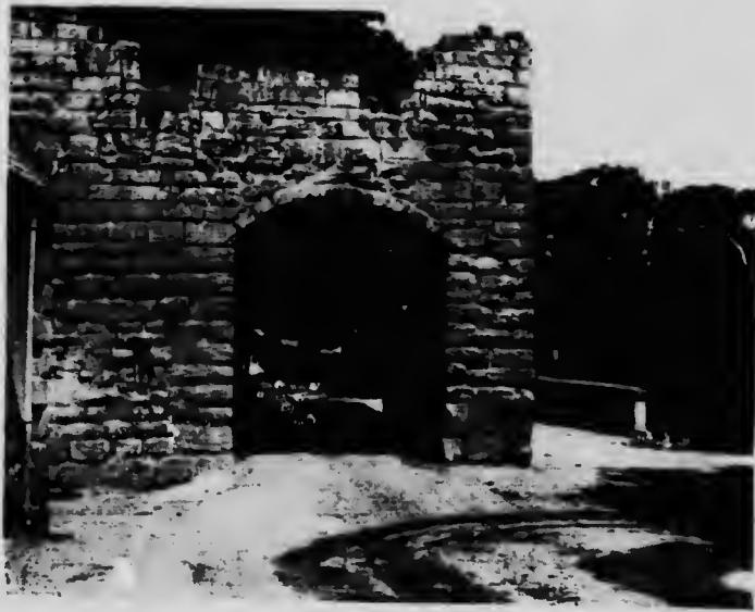
GATEHOUSE ON WARKWORTH BRIDGE.
